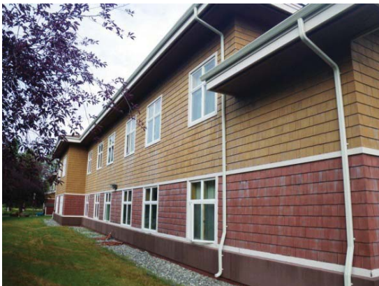
Worn Cedar Siding Paint on Building 7
